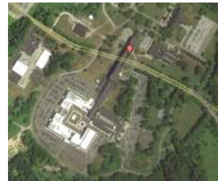
CoActiv's Primary Datacenter in New York
